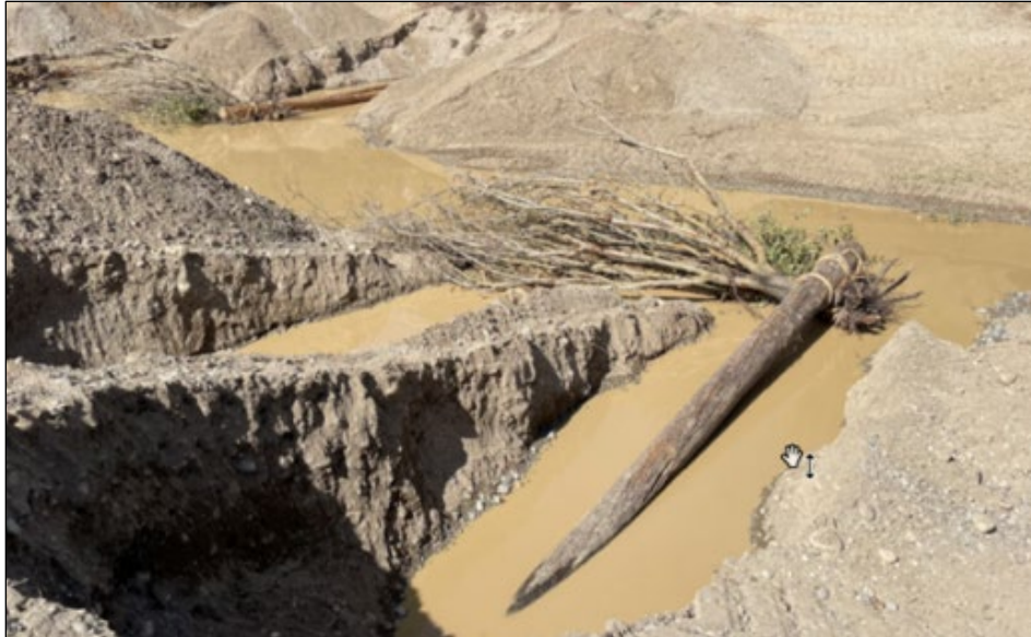
Figure 11: Habitat IWM Anchoring Example
